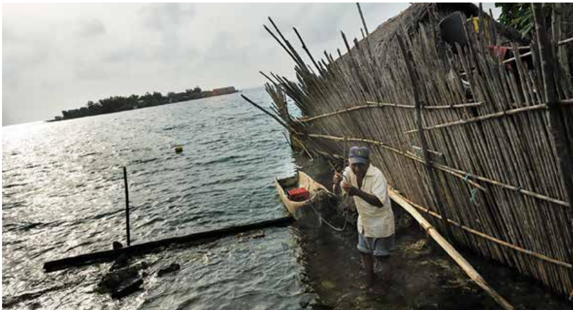
THESE SELF-MADE SEAWALLS IN GUNAYALA ARE NO MATCH FOR RISING SEA LEVELS AND EVER-WORSENING COASTAL EROSION. (IMAGE: KADIR VAN LOHUIZEN / NOOR)
